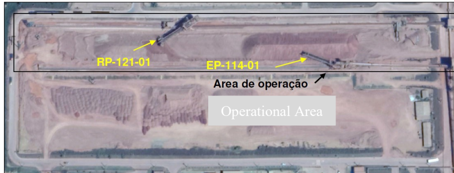
Figure 2. Bauxite homogenization yard at Hydro Paragominas.
